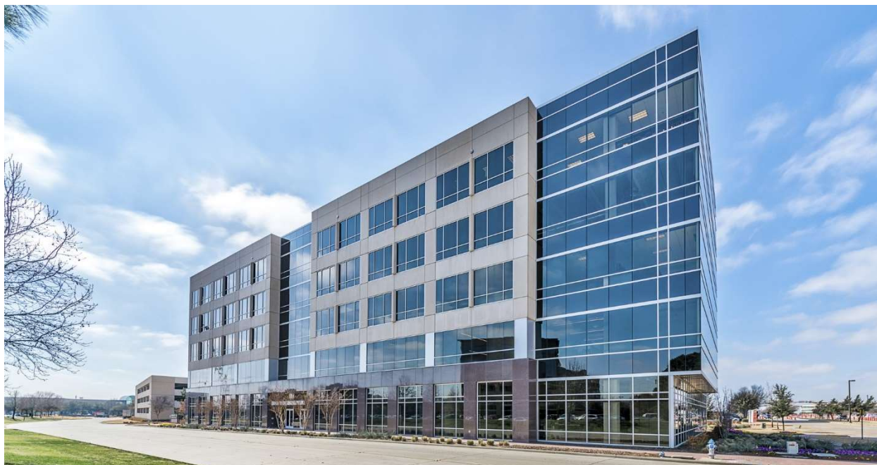
A partnership acquired the 130,371 square-foot Lincoln Legacy II building at 5810 Tennyson Parkway
